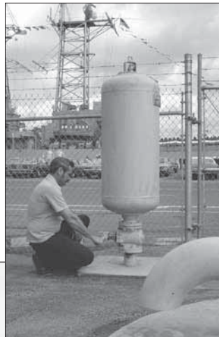
Refineries — Shock from pump starting and stopping
