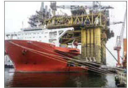
Synchronous superlift and launch
