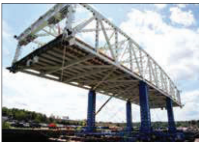
Incremental bridge lifting
