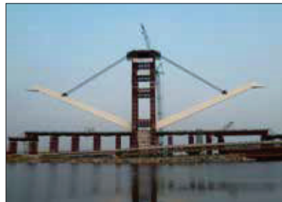
Jacking with high capacity precision control
