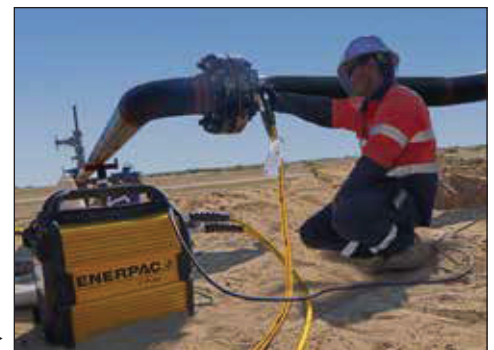
E-Pulse torque pump used for high volume fastening applications.
