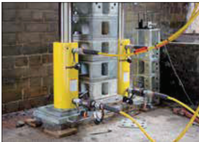
Bridge lifting and launching
