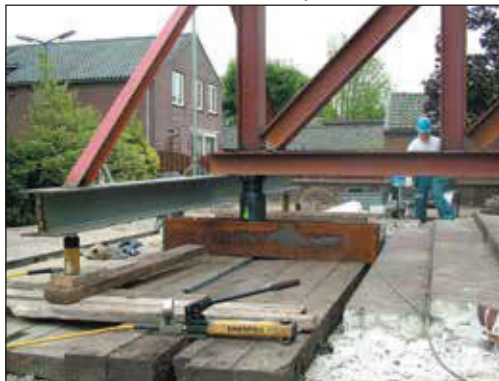
▼ P392 in action with RC256 cylinders.
