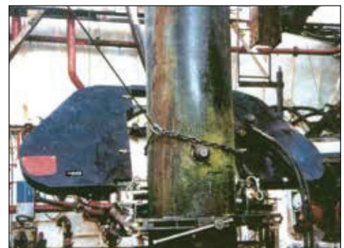
▼ Decommissioning job with band saw.
